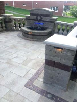
The masonry fence enclosing the patio consists of substantial stone balusters flanked by dry-stacked square columns. The columns are constructed with the Brussels Dimensional System with Brussels Fullnose coping, both in the Sandstone color option. A double band of Burnt Clay Copthorne pavers creates a consistent look between the masonry wall, water feature and patio.
